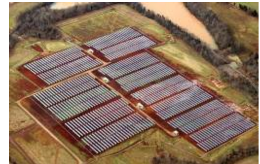
Duke Energy- 4 of 17MW, Cotton Grove, NC Crystalline panels, one axis, ground mount.
