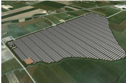
72 MW - Rovigo, Italy. Crystalline panels, fixed tilt, ground mount. Largest being built in Europe.
