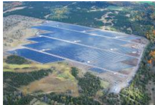
First Light – 9MW - Napanee, ON Thin film panels, fixed tilt, First Utility Scale- Canada
