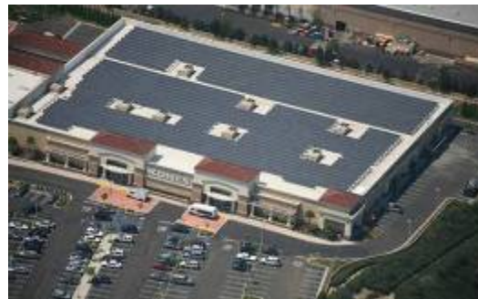
Kohl's - 409 KW - Laguna Niguel, CA Crystalline panels, fixed tilt, roof mount.
